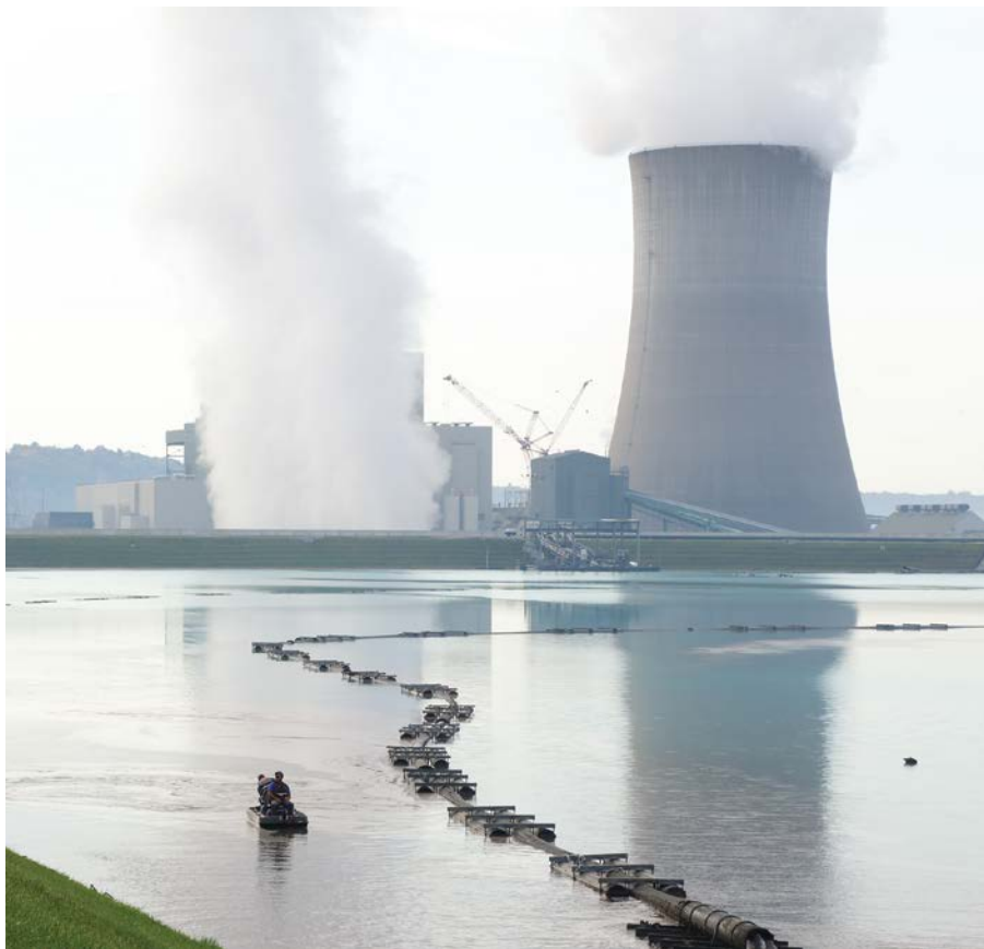
Trimble County Generating Station
